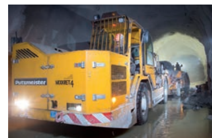
Concrete transport and mixing
